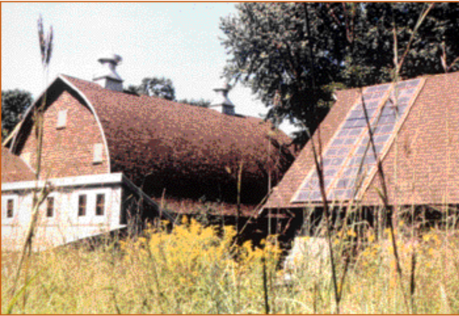
This nature center near Cedar Rapids, IA, uses solar electricity to run low-wattage, energy-efficient lights.
